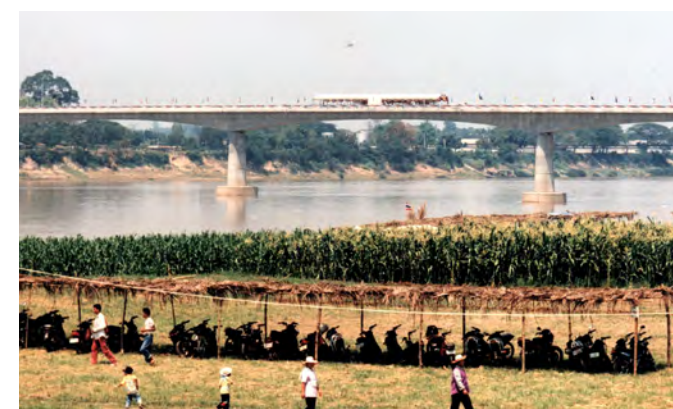
A tent was erected in the middle of the First Lao-Thai Friendship Bridge for the opening ceremony on 8 April 1994.
